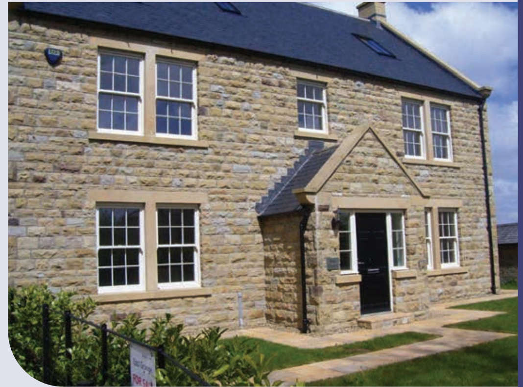
Image 7.12: An example of good window design on modern development.
