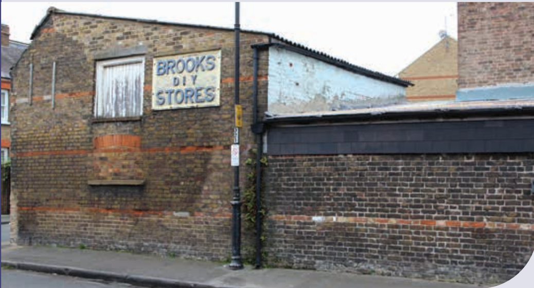
Image 7.8: An inactive frontage with no openings at street level.
