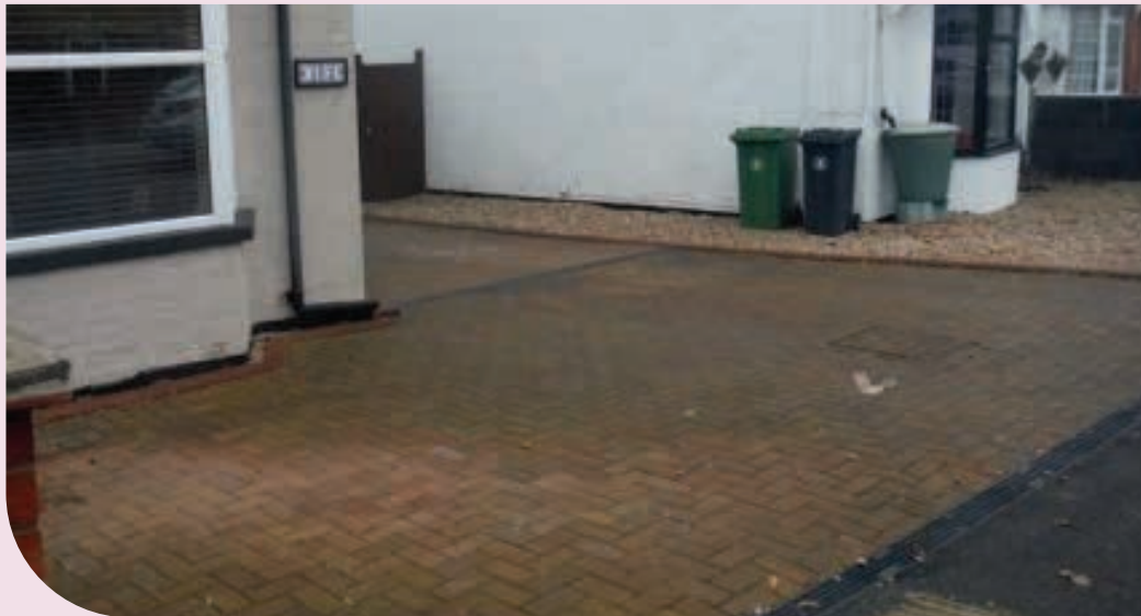
Image 9.5: Hardstanding area that dominates the front of the property and has resulted in the loss of soft landscaping and plot enclosure.
