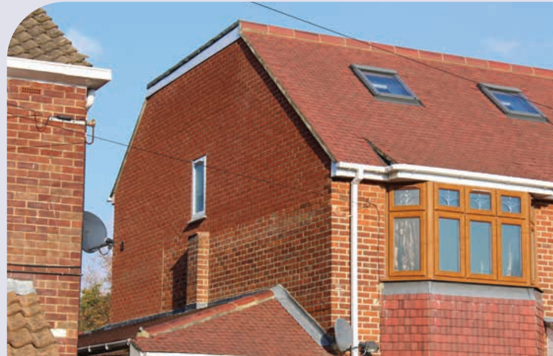
Image 7.5: Example of poor roof design with unattractive bridging flat roof section, awkward angles and poor treatment to top of bay window.
