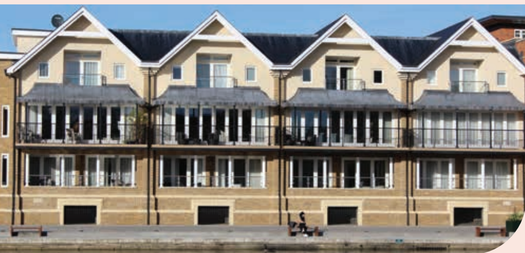
Image 11.2: A high quality design that has raised floor levels and provided void space in a visually pleasing and historically sensitive manner.
