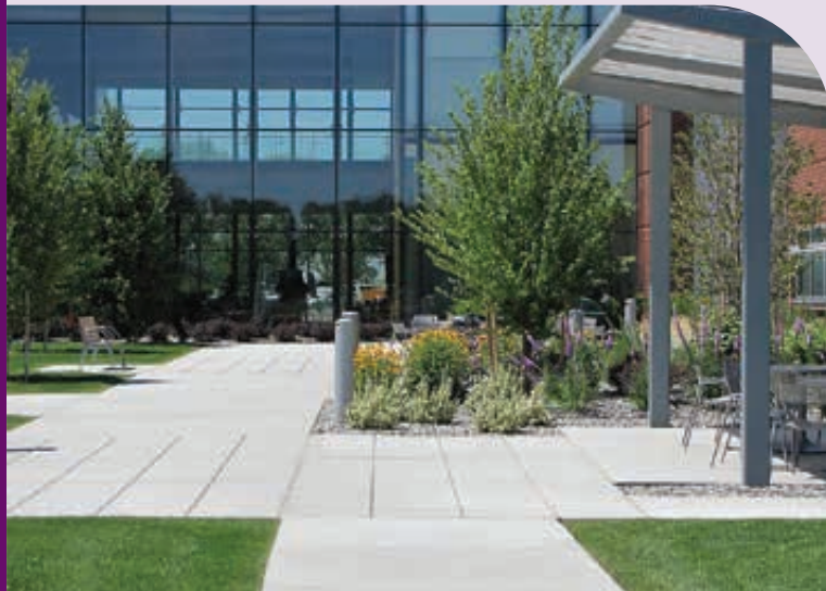
Image 8.6: Sunny outdoor amenity space for workers with green infrastructure and good facilities for sitting and eating outside.
