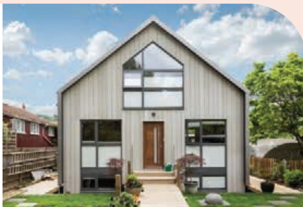
Figure 11.1 Innovative example of a floating house that floats itself upwards to escape flooding on the River Thames. Marlow, Buckinghamshire by Baca Architects.
