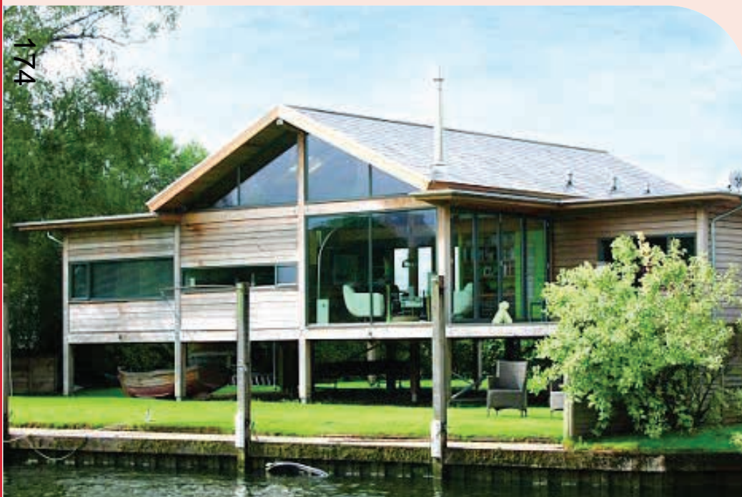
Image 11.3: Contemporary example with the ground floor raised above flood levels of the floodplain. This clearly distinguishes the living areas from the floodzone, by raising the house on stilts.
